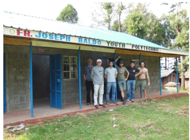
The Polytechnic (professional workshop) construction
